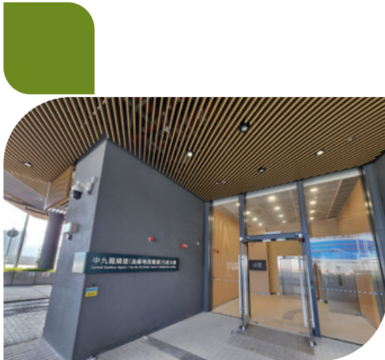
Central Kowloon Route – Building, electrical and mechanical works – Design, supply and installation of suspended ceiling system 中九龍幹線－大樓及機電工程－設計、供應及安裝假天花系統
