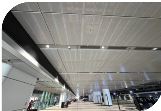
HKIA Terminal 2 Expansion Works – Design, supply and installation of lower-level baffle and external ceiling system 香港國際機場二號客運大樓擴建工程—設計、供應及安裝低層天幕及室外天花系統
