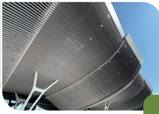
HKIA Terminal 2 Expansion Works – Design, supply and installation of lower-level baffle and external ceiling system 香港國際機場二號客運大樓擴建工程—設計、供應及安裝低層天幕及室外天花系統
